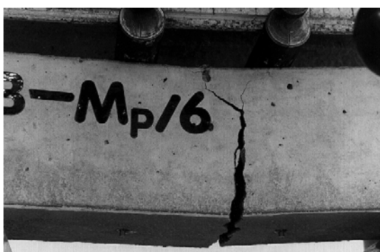
Fig. 5. Image of destruction of a beam covered with the PCP-1 coating tested after twenty five cycles of freeze resistance
