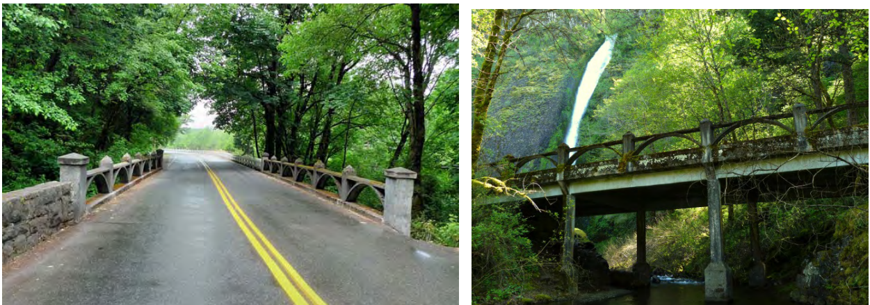
Figure 1: The Horsetail Creek Bridge
